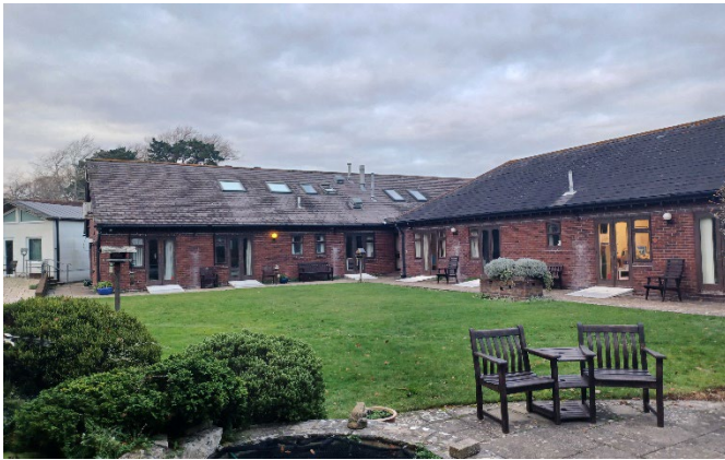
Existing IPU building
