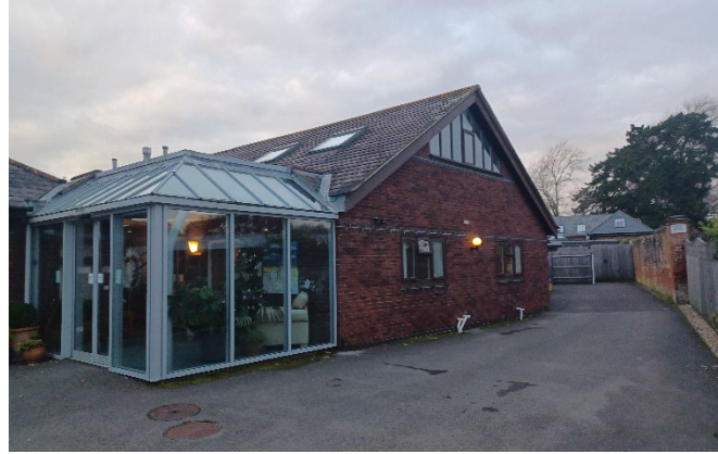
Existing IPU building
