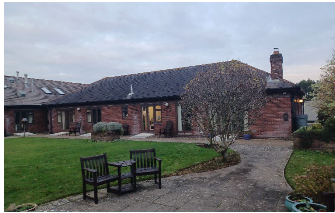
Existing IPU building
