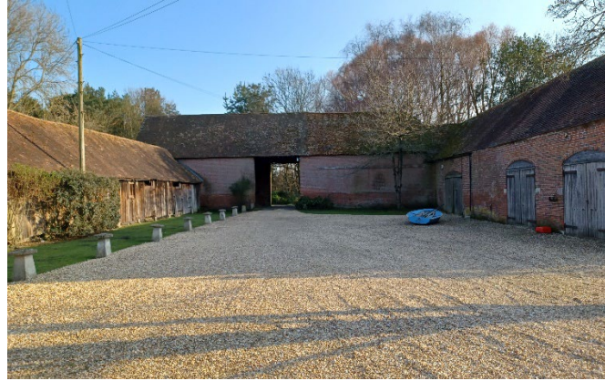
Courtyard looking to the South
