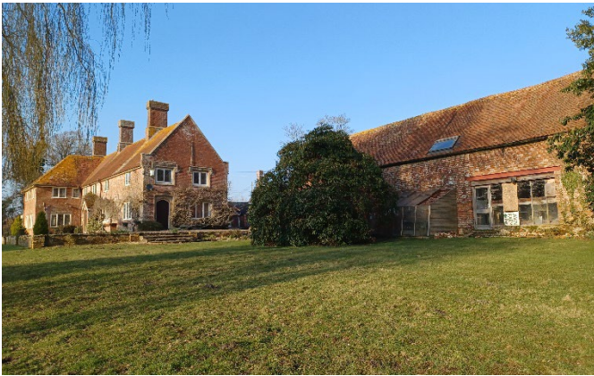
Rear view of severance
