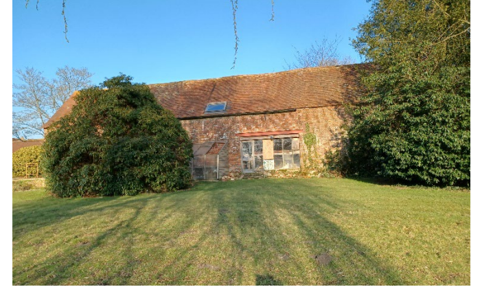
West Range Barn (West Elevation)
