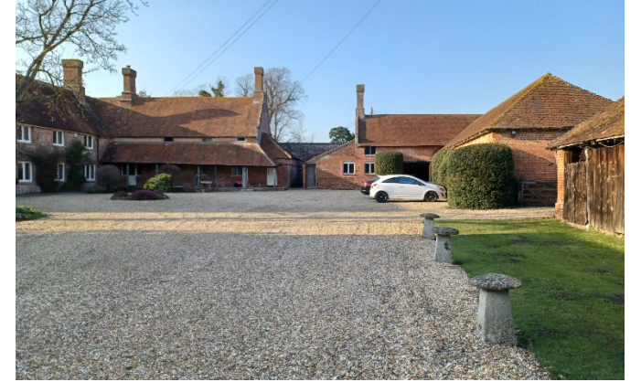
Courtyard looking to the North
