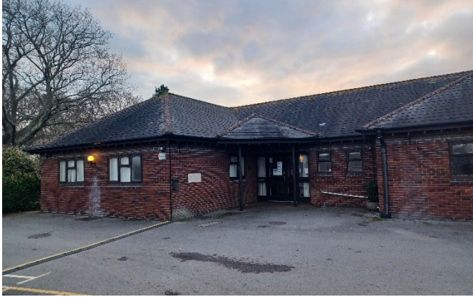
Existing IPU building
